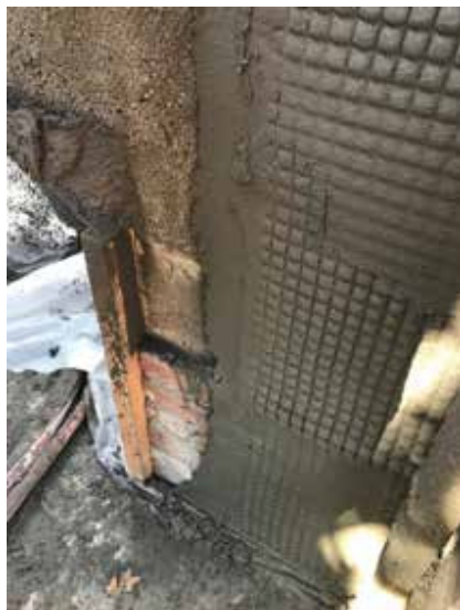
Figure 4. FRCM fabric being installed into matrix.
