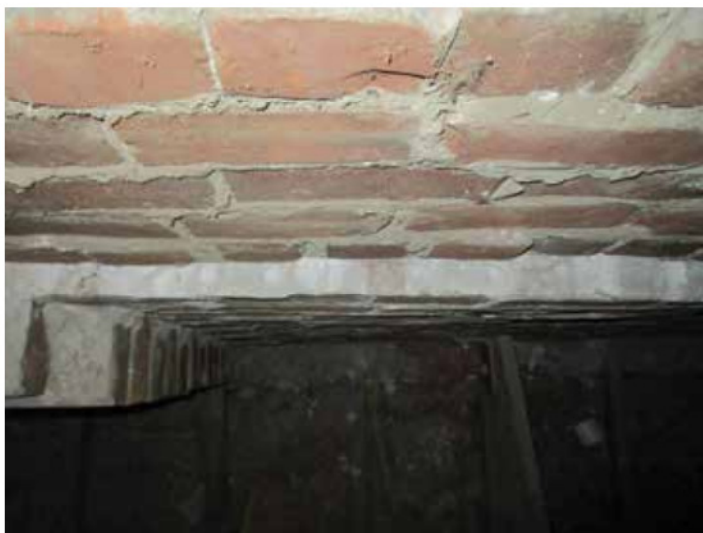
Figure 3. Horizontal offset of brick in the attic.
