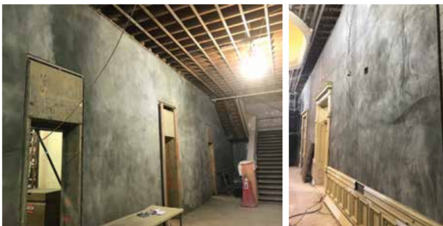
Figure 6. Finished FRCM installation on first floor (left), second floor (right).
