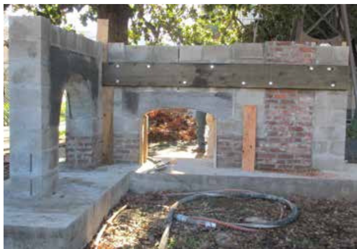
Figure 3. Mockup prior to installation of FRCM.
