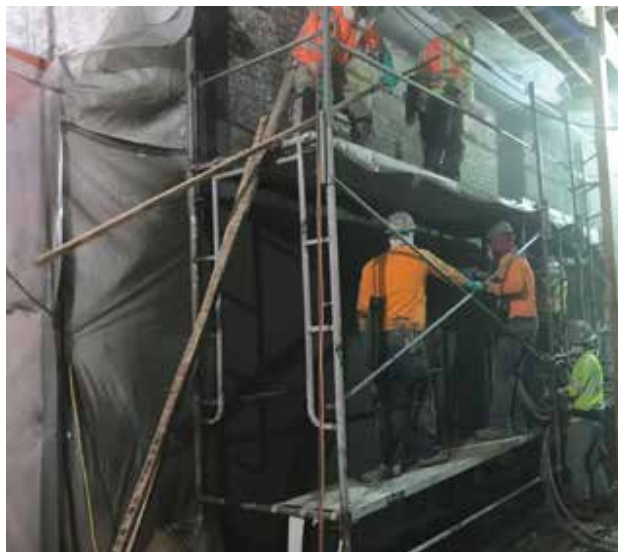
Figure 5. FRCM installation.
