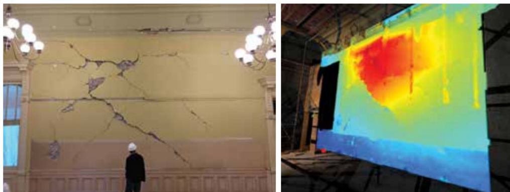
Figure 5. Site photo of damaged wall and heat map showing offset.
