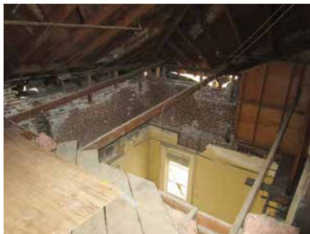
Figure 2. Courtroom view from the attic where brick partially collapsed the ceiling below.
