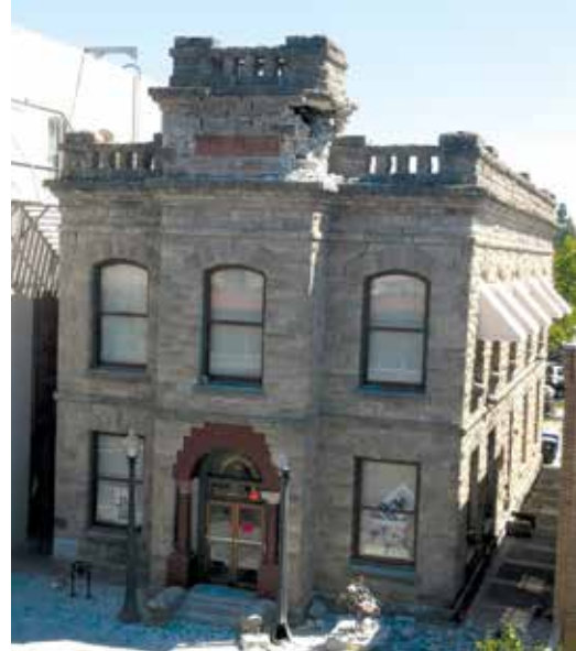
Figure 1. Library after the earthquake.
