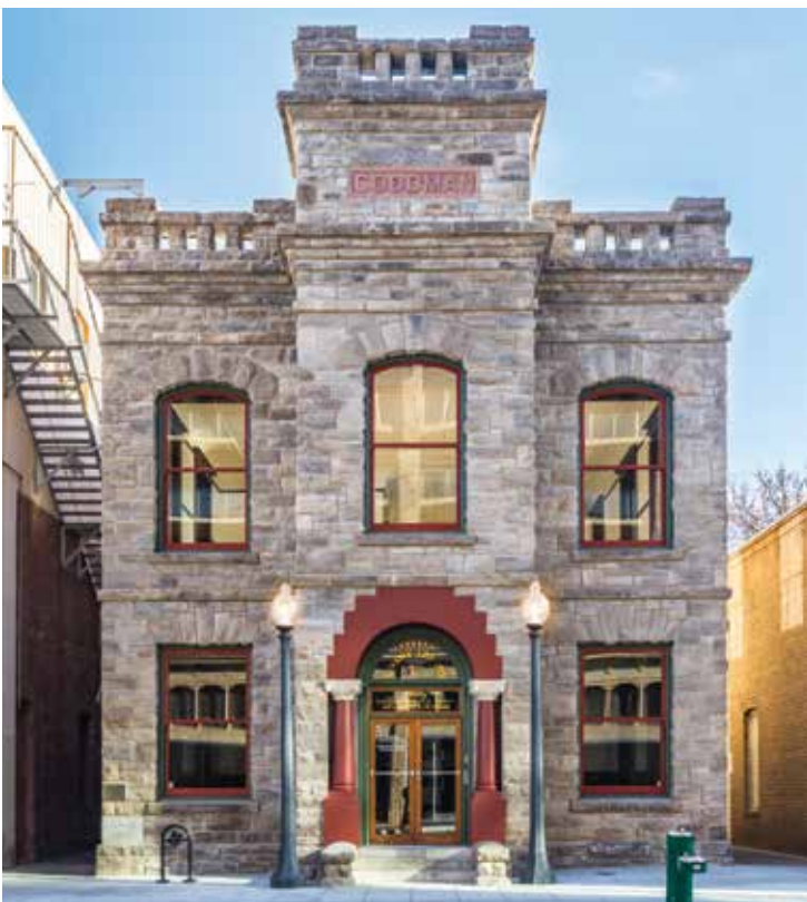
Restoration of the Goodman Library completed December 2017. Courtesy of Justin Lopez Photography.
