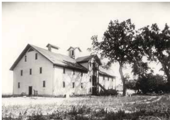
Figure 1. Historic Trefethen Winery building (Eshcol Winery c 1915). Courtesy of Trefethen Family Vineyards.
