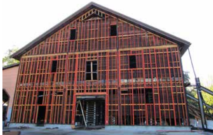
Figure 5. Retrofitted gable end wall framing.
