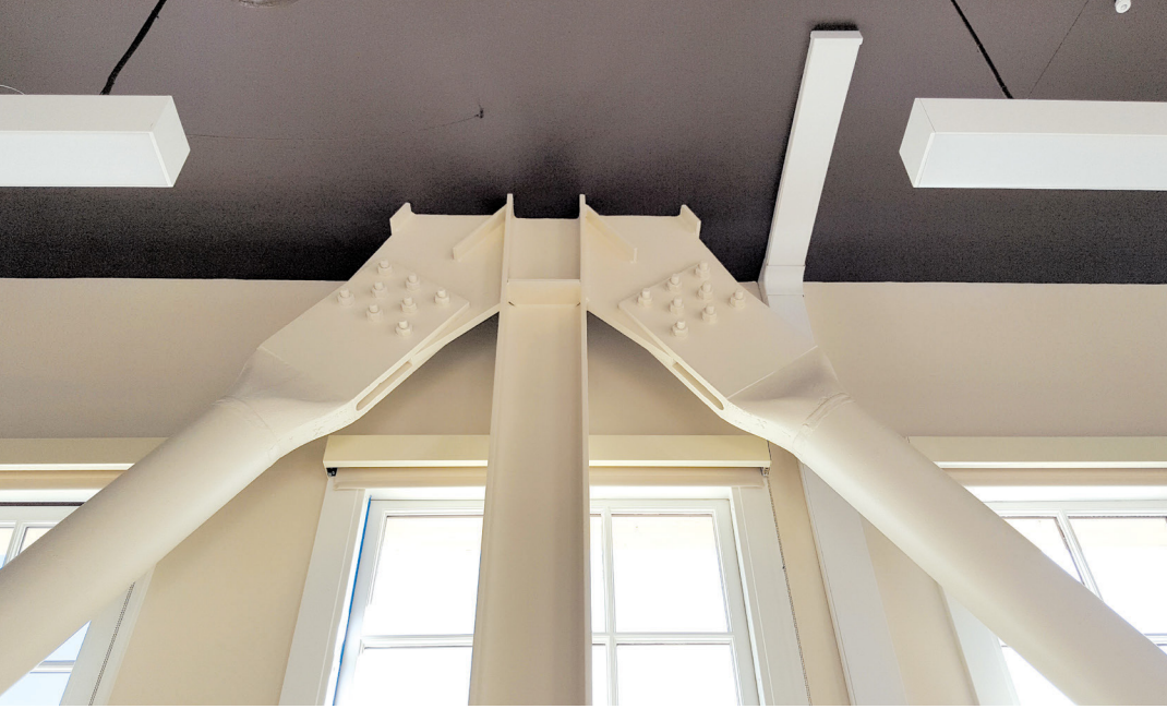
Cast Connex HSC brace connection.
