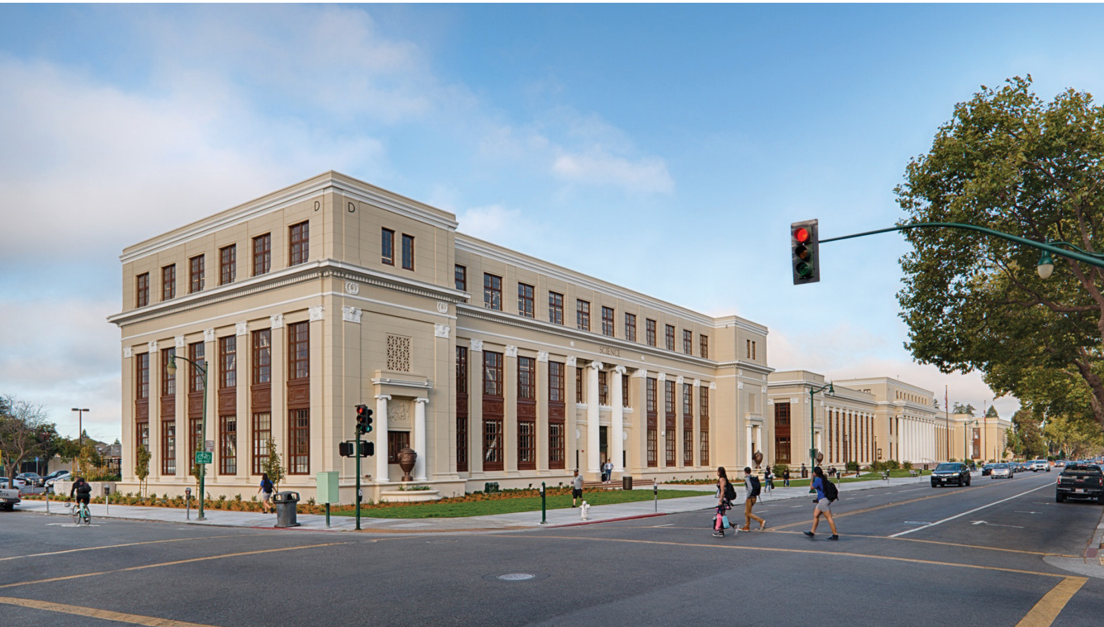
Looking down Central Avenue.
