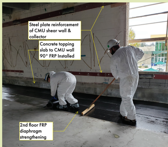
Fig. 5. Steel plates were used for CMU wall shear wall and collector strengthening. FRP diaphragm strengthening is installed by unrolling epoxy-saturated fabric.
