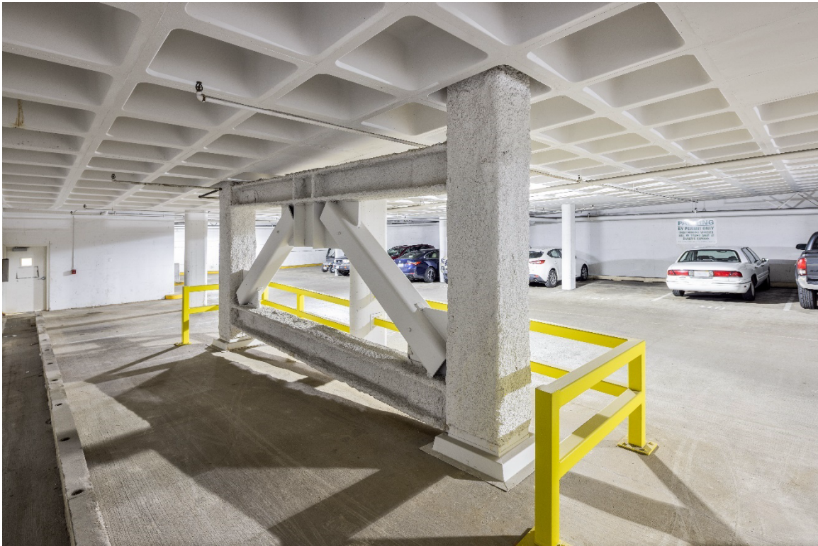
Figure 15: Braced Frame Installed at the Lowest Level of the Parking Garage
