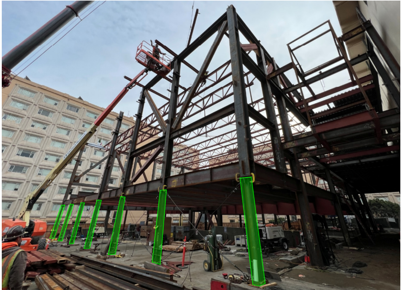
Figure 24: Temporary Shoring Posts (Green) To Support Long-Span Truss During Erection
