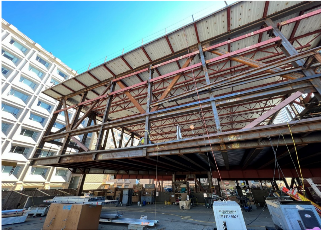
Figure 7: North Elevation Showing Truss A During Construction
